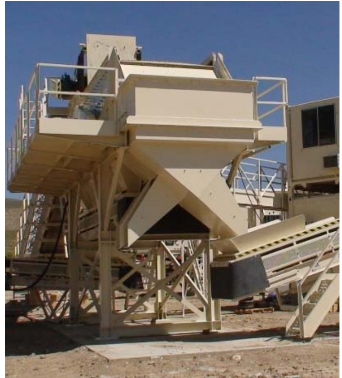
Firstgold's primary crusher at the Relief Canyon mine site
