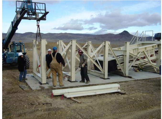
Base of the crusher being erected.
