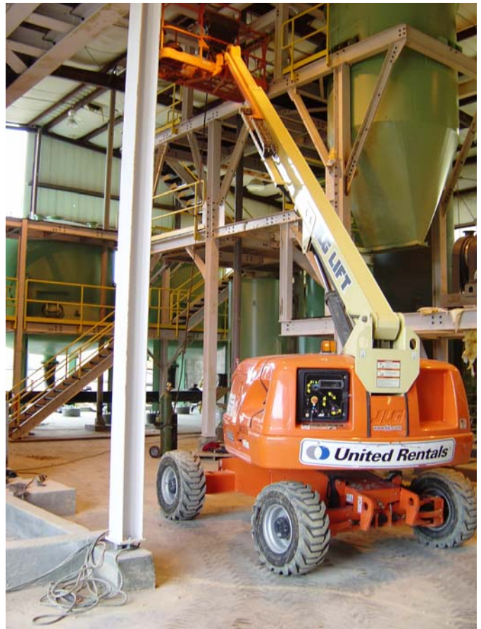
Crews work to install scaffolding.
